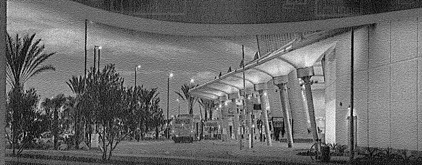
San Diego Int'l Builds Consolidated Rental Car Facility
